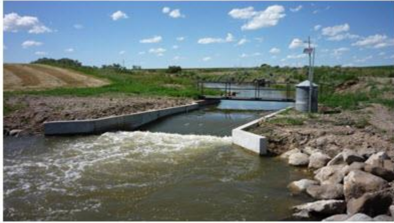
Fig. 19.8. Repleg flume or long-throated flume. (Source: http://inmtn.com/images/flumes/bench-b-ramp-flume.jpg )
